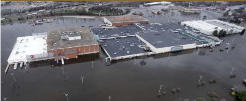
Warwick Mall overtaken by the Pawtuxet River - Warwick, RI at 1030 am Wednesday 3/31/10. Photo: RI ANG
