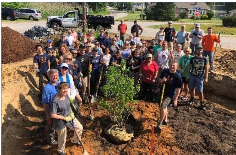
Rain gardens, like this one at the Community Hall, can help reduce street flooding. Photo by ERICD
