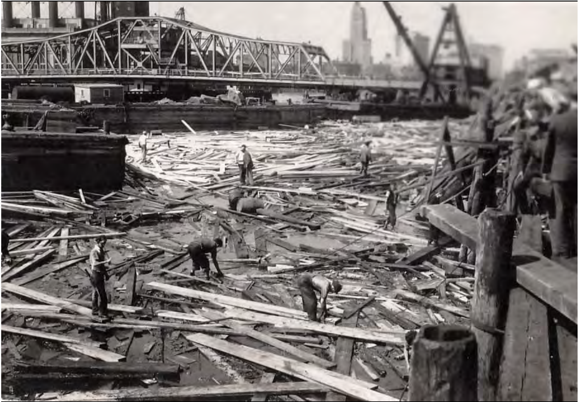
Point Street Bridge, Providence, 1938
